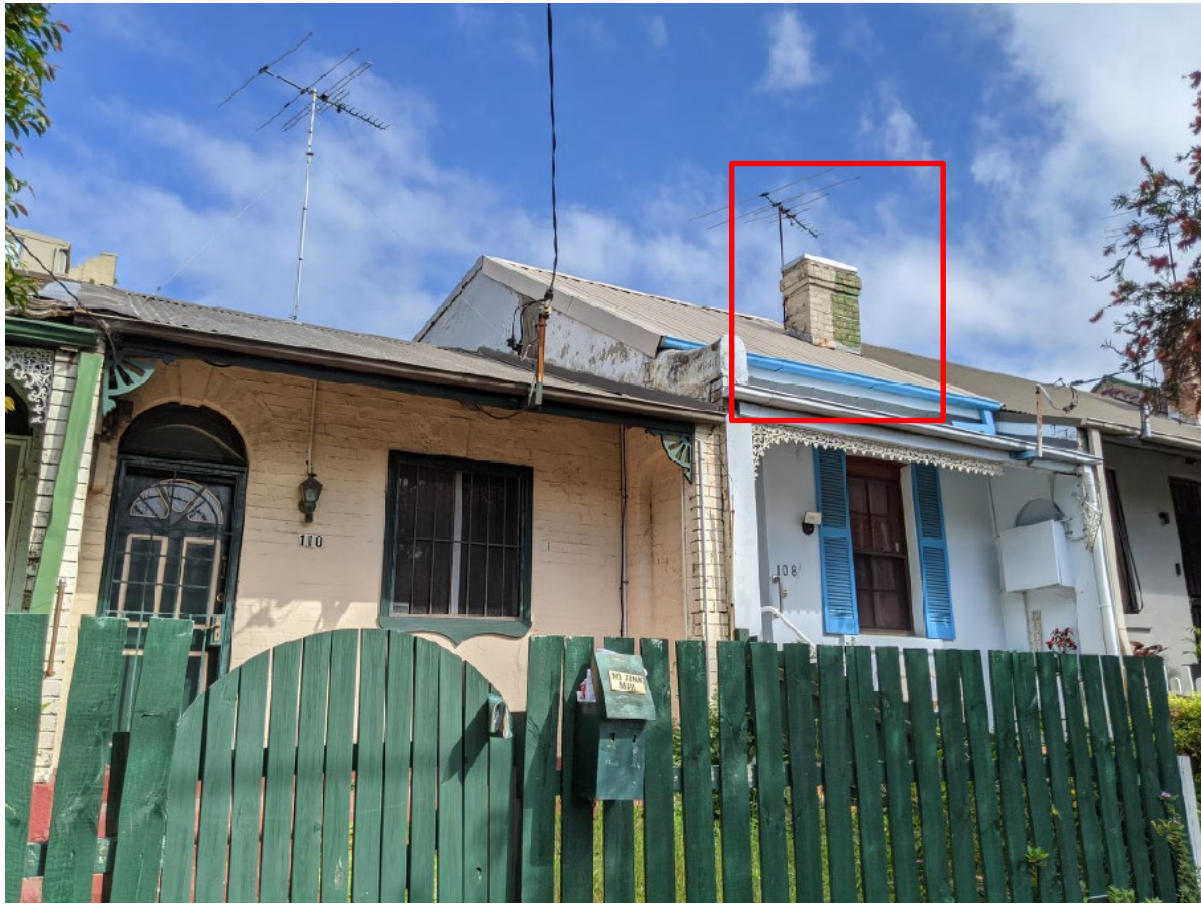
shared chimney of 106 and 108 Victoria St
