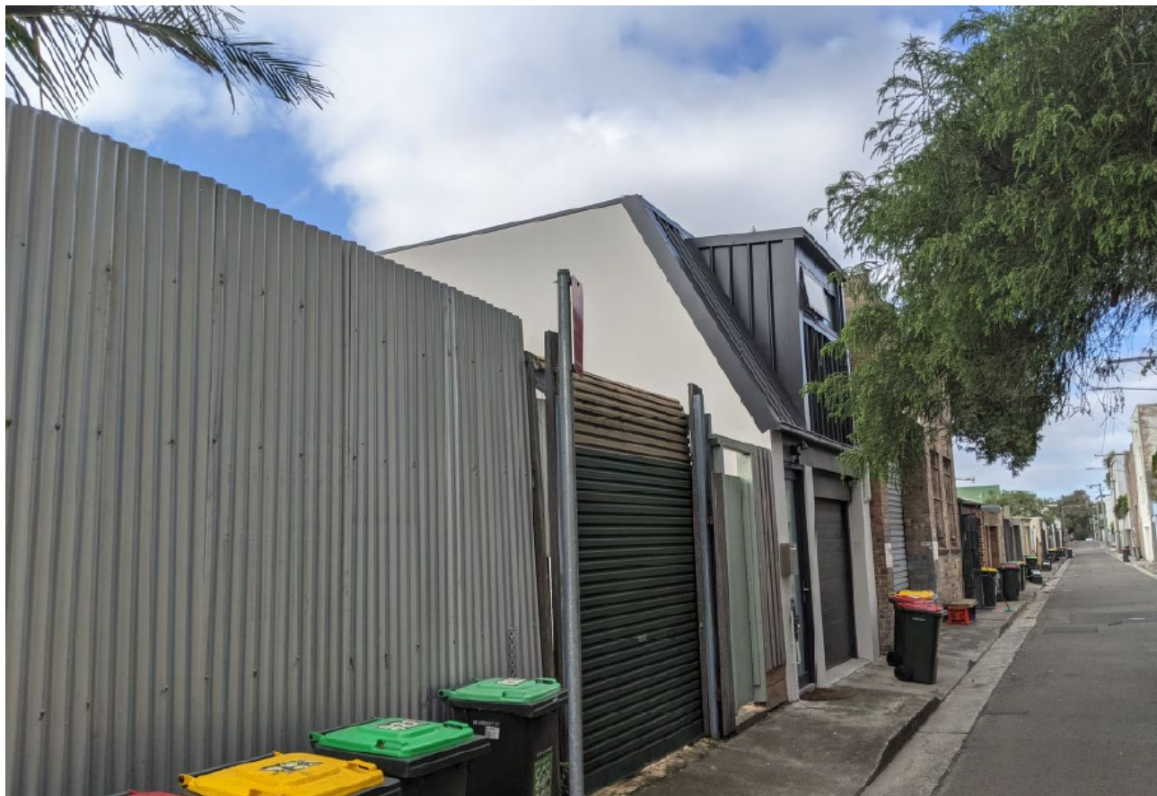
laneway structure at 122 Victoria St
