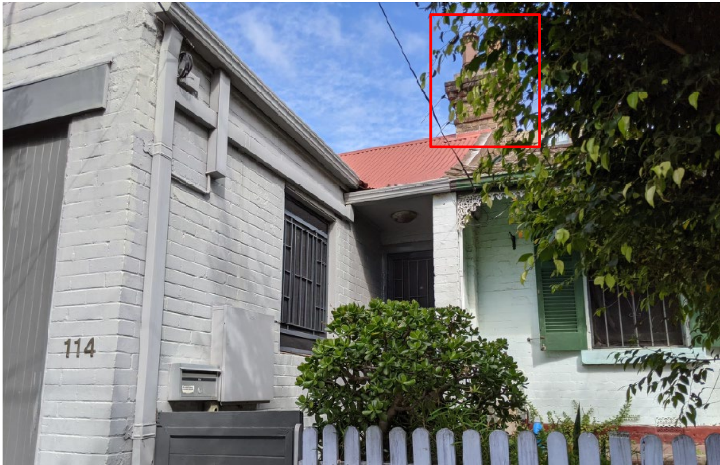
shared chimney of 112 and 114 Victoria St
